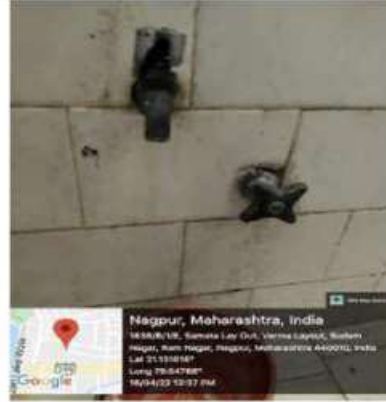
Cocks to be replaced by push buttons
