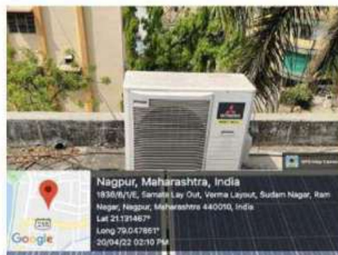
AC Condensers exposed to direct sunlight
