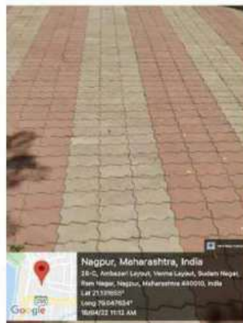
Cement blocks in college for Water Harvesting
