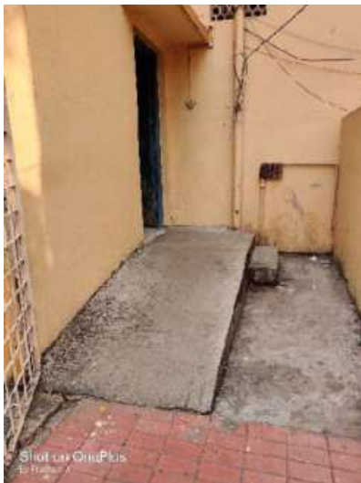
Divyangjan Friendly Ramp for Urinals
