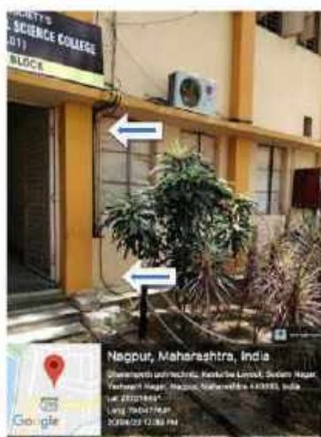
AC Condensed Water given to plants
