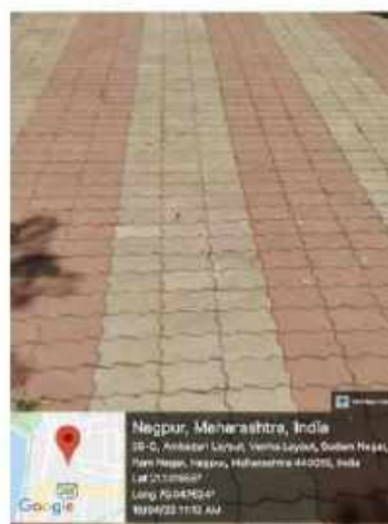
Cement blocks in college for Water Harvesting
