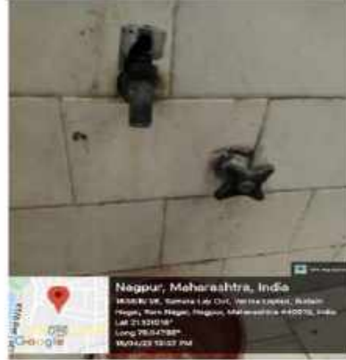
Cocks to be replaced by push buttons
