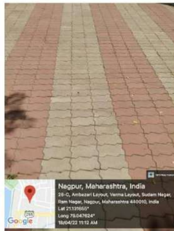
Cement blocks in college for Water Harvesting
