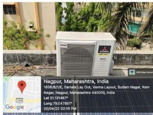
AC Condensers exposed to direct sunlight
