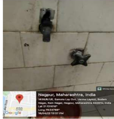
Cocks to be replaced by push buttons
